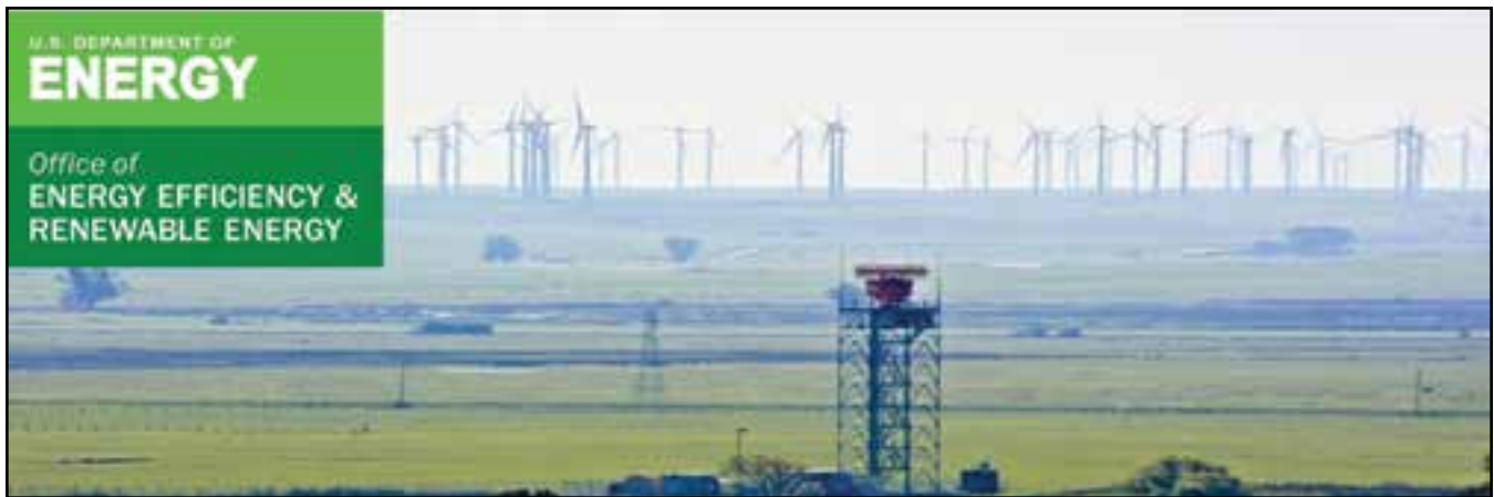
Wind turbines located near radar systems can degrade the air surveillance picture. Photo of Travis Air Force Base, California. Photo credit: Bryan Miller
