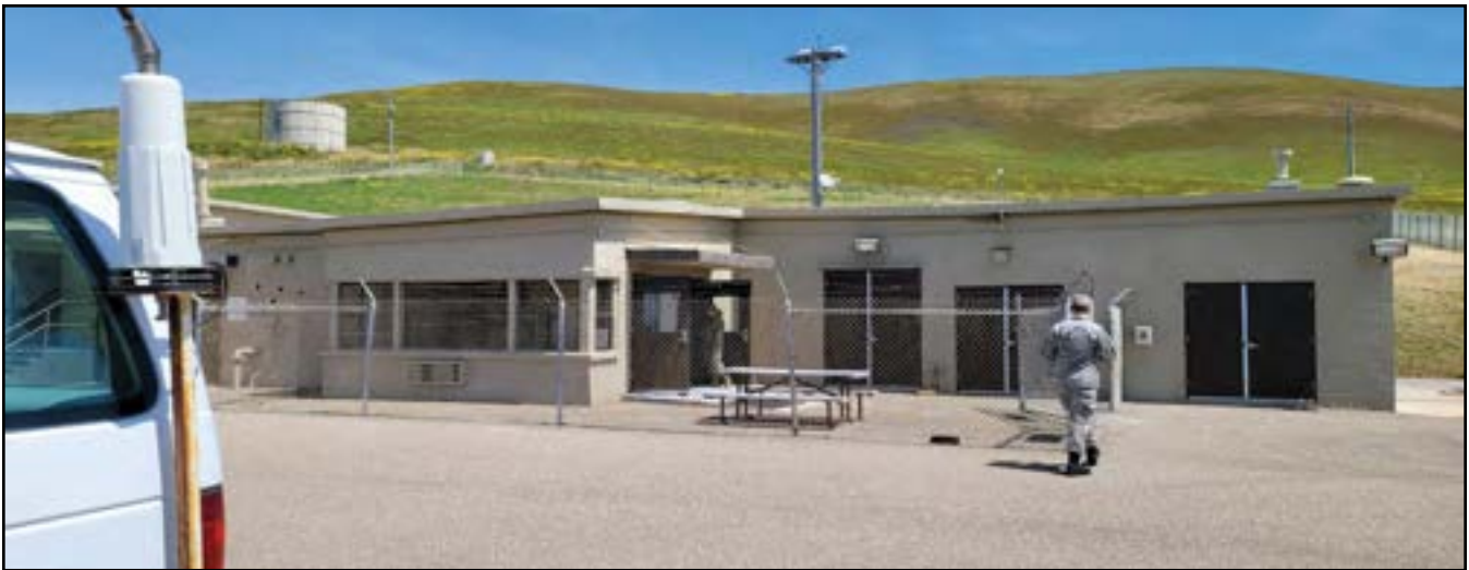
Above ground, the entry to the underground bunker complex for the ICBM Minuteman III test missile launch facility is a simple looking building. Photo credit: Maj. David Andrews
